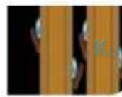
Condensation water washes away the dust and grease
