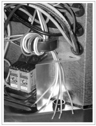
Figure 5. Low Voltage Compartment Control Wiring Connections
